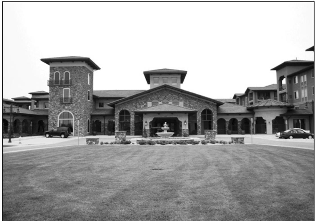
Work will be completed in the next 60 to 90 days on the final phase of development of the Terracina Villas apartments in Broomfield.
